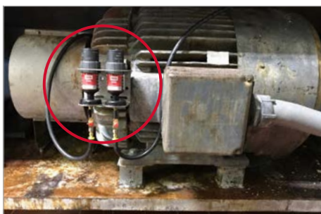
Remote bearing lubrication on an electric motor
